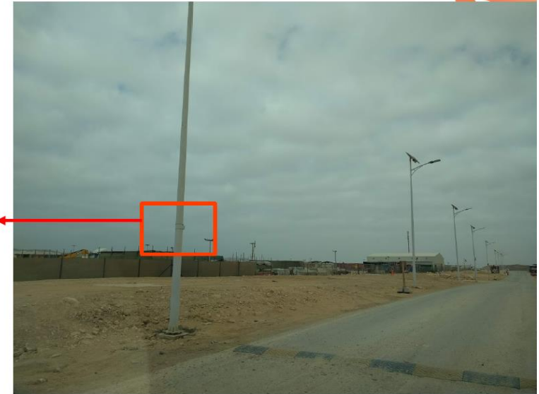
Bluetooth beacons hooked near to a speed hump to detect entry / exit by car
