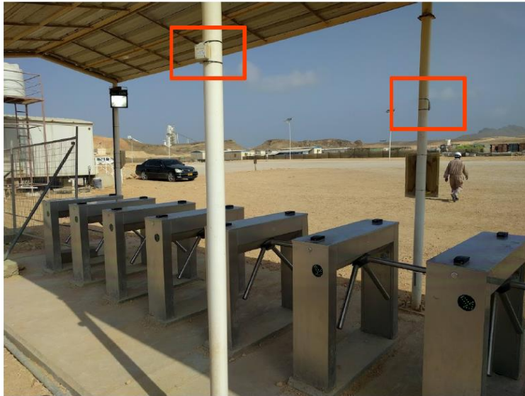
Bluetooth beacons hooked near turnstiles to detect walking site entry / exit
